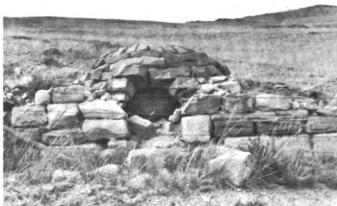
FIGURE 8.—First coke oven in Montana, built in 1881 by W. H. Williams in the SE \frac{1}{4} SW \frac{1}{4} sec. 24, T. 2 S., R. 8 E., Livingston coal field. The oven is made of blocks of sandstone from the Cokedale and Eagle Formations.
