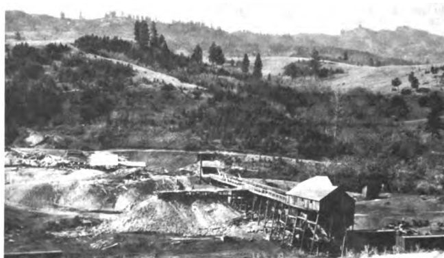
FIGURE 12.—The Maxey Bros. No. 1 mine portal and tipple, Livingston coal field. Wooded hills in background are underlain by Eocene conglomerate and volcanic breccia. Chimney Rock shows on skyline on right side of photograph. View is to the west. Photographed by W. R. Calvert in 1908.
